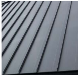
Timberline HDZ 30 yr Arch Shingles - Charcoal Shed Dormers only. Metal Hidden Rib Fastener Roofing - Midnight Black Front Mono-Slope and Covered Porches.
