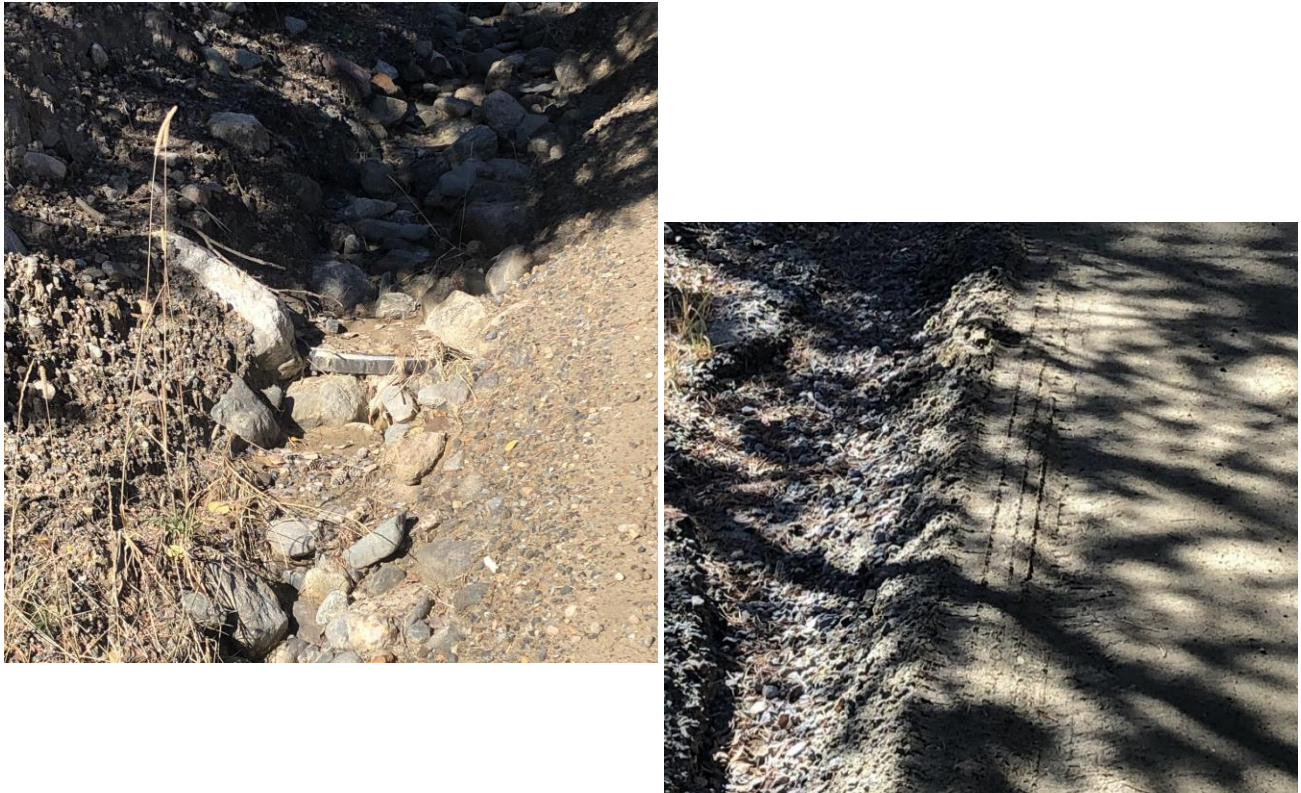
Figure 3 – Longitudinal Drainage Conditions
