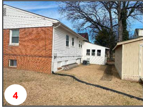
Figure 2.7.1.5 Property #7: Back (east side)
