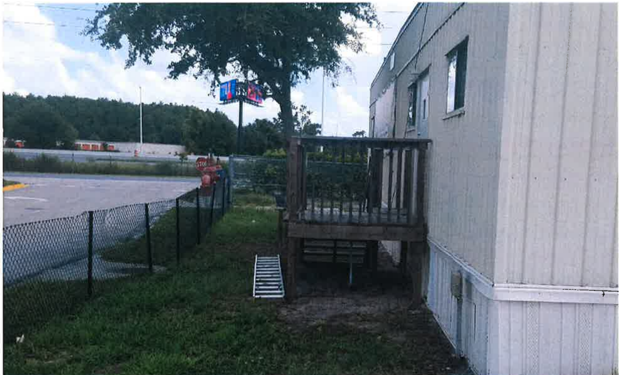
Office Side Street Setback from Street Right of Way
