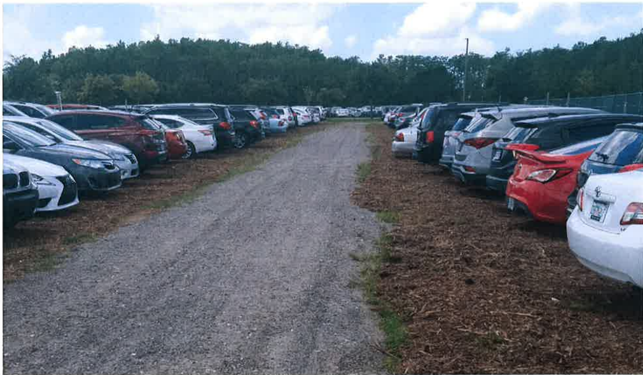
Milling Drive Aisle With Mulch Parking Spaces
