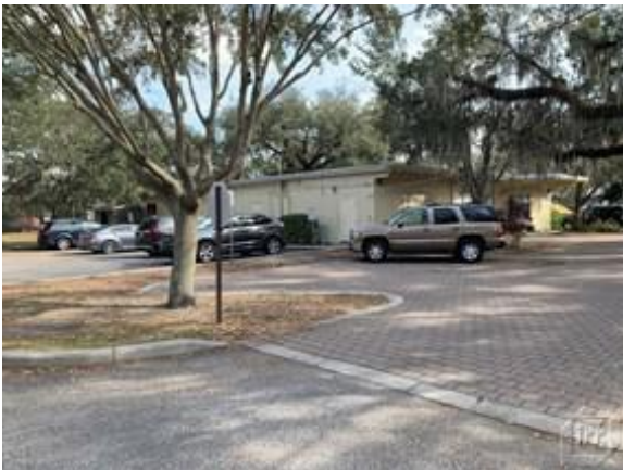
An exterior view of the field house. (Photograph taken on February 10, 2021)
