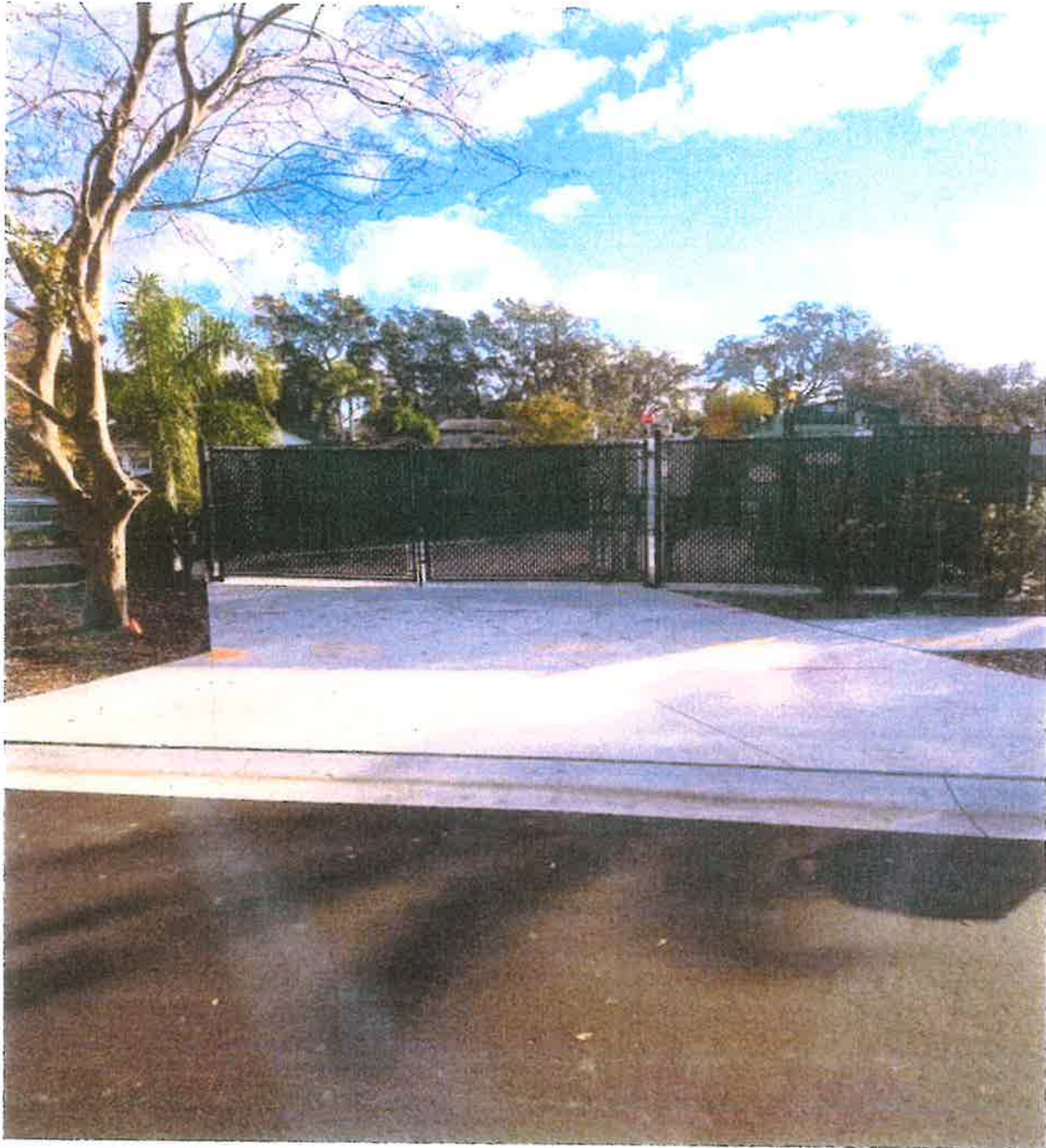
The new lift station
