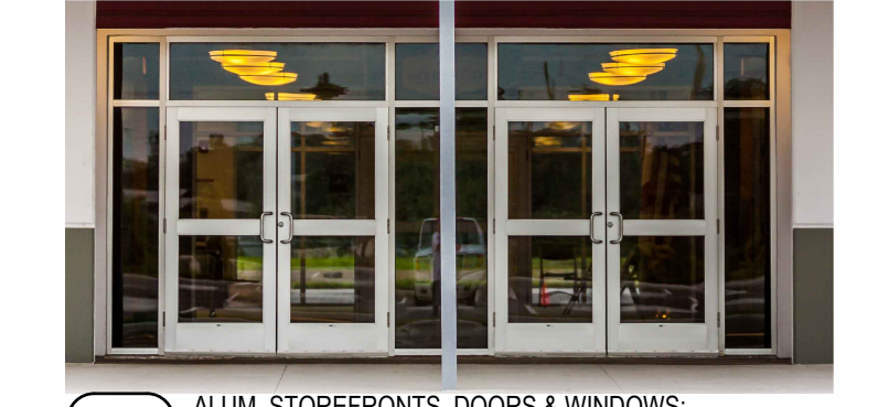
M-3 ALUM. STOREFRONTS, DOORS & WINDOWS: ANODIZED ALUMINUM W/ SOLAR-E PLUS GREY GLASS
