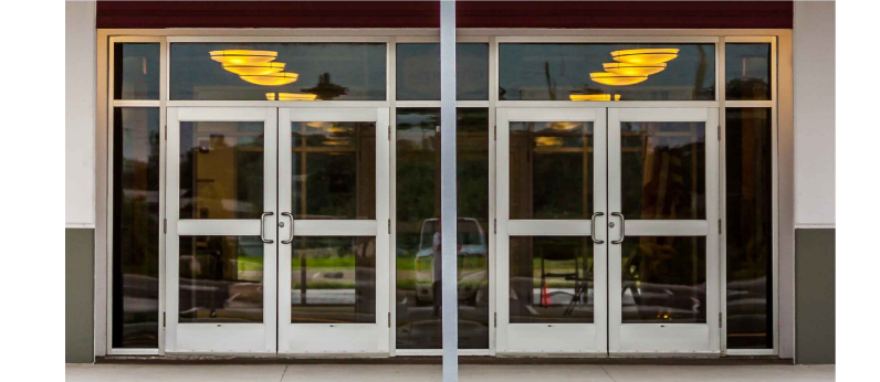
M-2 ALUM. STOREFRONTS, DOORS & WINDOWS: ANODIZED ALUMINUM W/ SOLAR-E PLUS GREY GLASS
