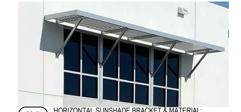
M-6 HORIZONTAL SUNSHADE BRACKET & MATERIAL: CLEAR ANODIZED ALUMINUM (SILVER)
