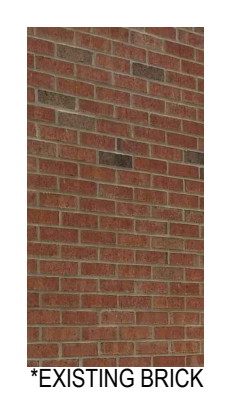
M-2 EXISTING BRICK
