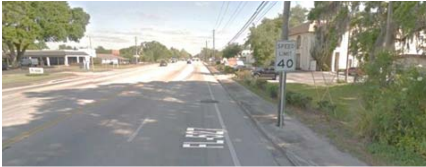
Existing Sidewalk Conditions/Obstruction
