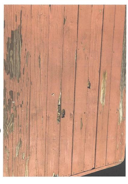
Boat cleats pulled out rotten wood, will be replaced with short posts for tie off
