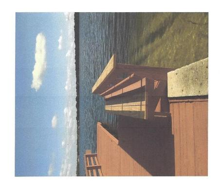
Years of weathering causing wood rot and paint checking
