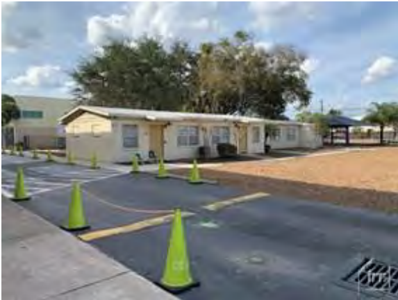
An exterior view of the classroom buildings. (Photograph taken on February 10, 2021)
