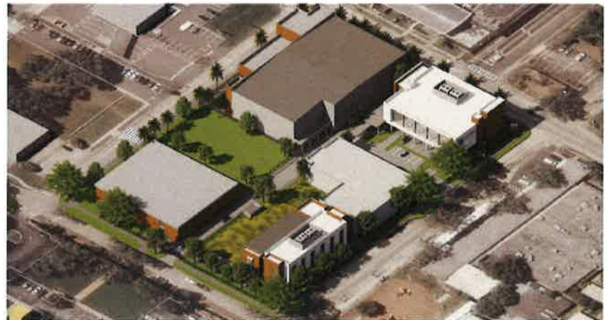
VIEW LOOKING SOUTHWEST SCALE: N.T.S. 1/2021
