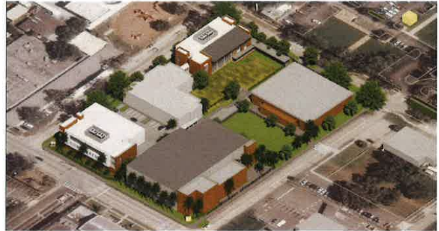
VIEW LOOKING NORTHEAST SCALE: N.T.S. 1/2021
