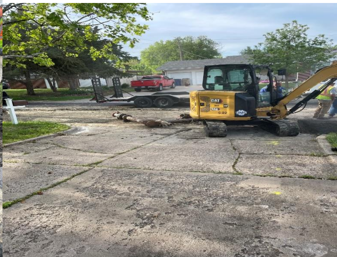
8" main at 4801 Kenawee a new valve and Fire Hydrant was installed at this location on 4/29/25
