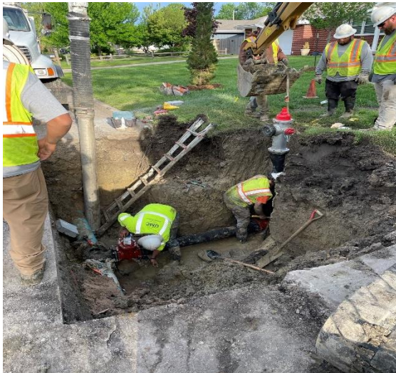
8" main at 4801 Kenawee a new valve and Fire Hydrant was installed at this location on 4/29/25
