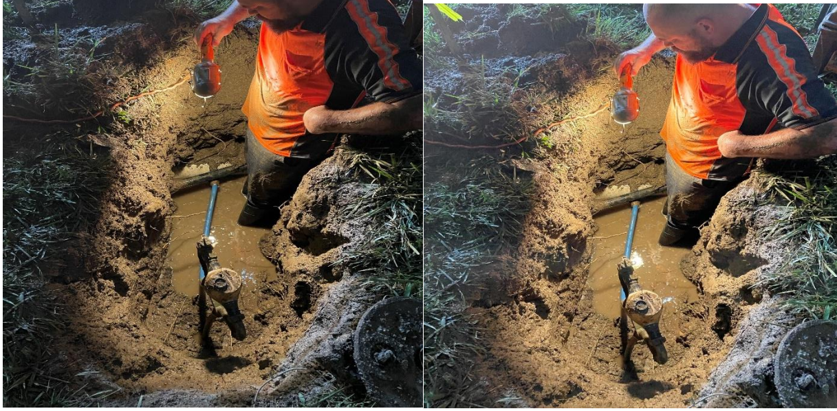
Service line repair at 5613 48 th street Circle
