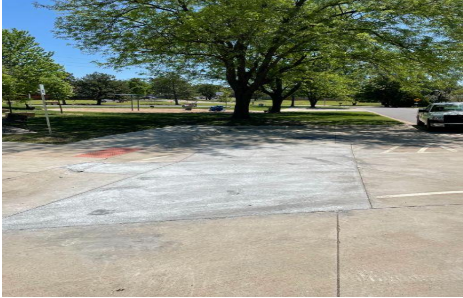
Bel Aire Park concrete repair
