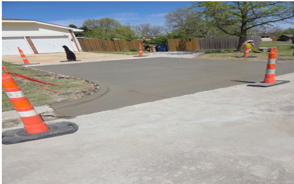
4335 Belmore driveway repair
