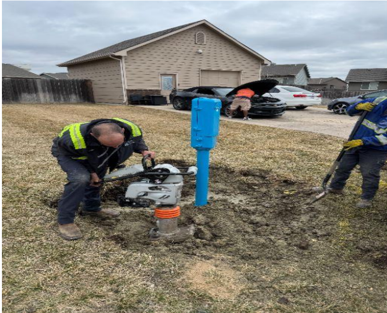
Sample Station installation
