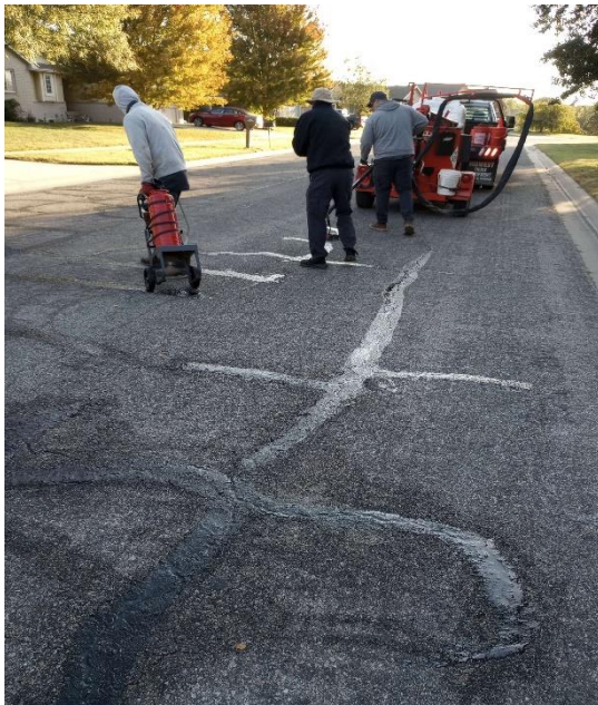
10/15/24 Quail Ridge crack sealing.
