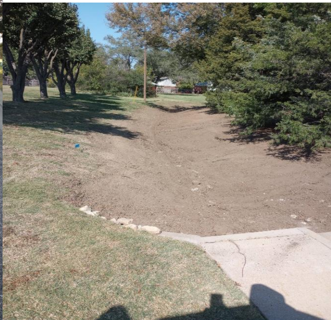
Tributary -7 regrading for drainage.
