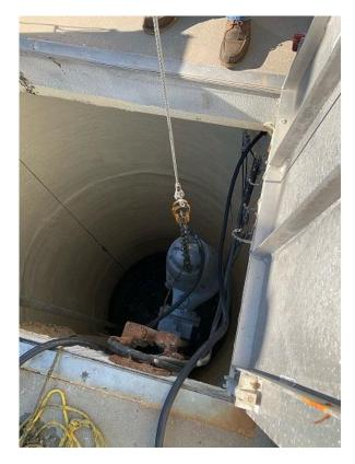
On the 25<sup>th</sup> staff received a high level alarm at the 53<sup>rd</sup> St. lift station and after inspection it was determined that the PLC (Programmable logic controller) unit failed. So the pumps were not working in automatic mode as they should. Staff had a portable pump brought in to keep the wastewater at a safe level. The new PLC was shipped overnight and replaced the next day and everything is operating as expected.
