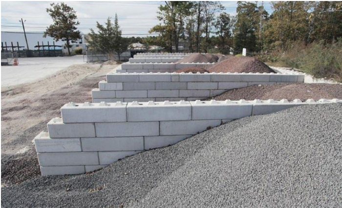
Bulk Material Storage - Concrete Bin Block
