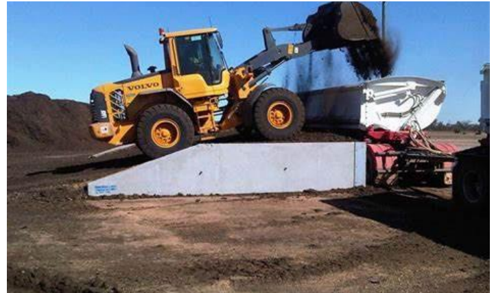
Material & Implement Loading Ramp
