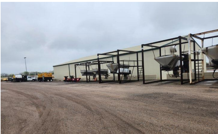
Salt Spreader Racks
