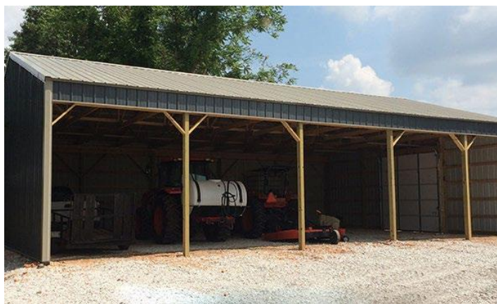
Open-Sided Pole Barn Storage
