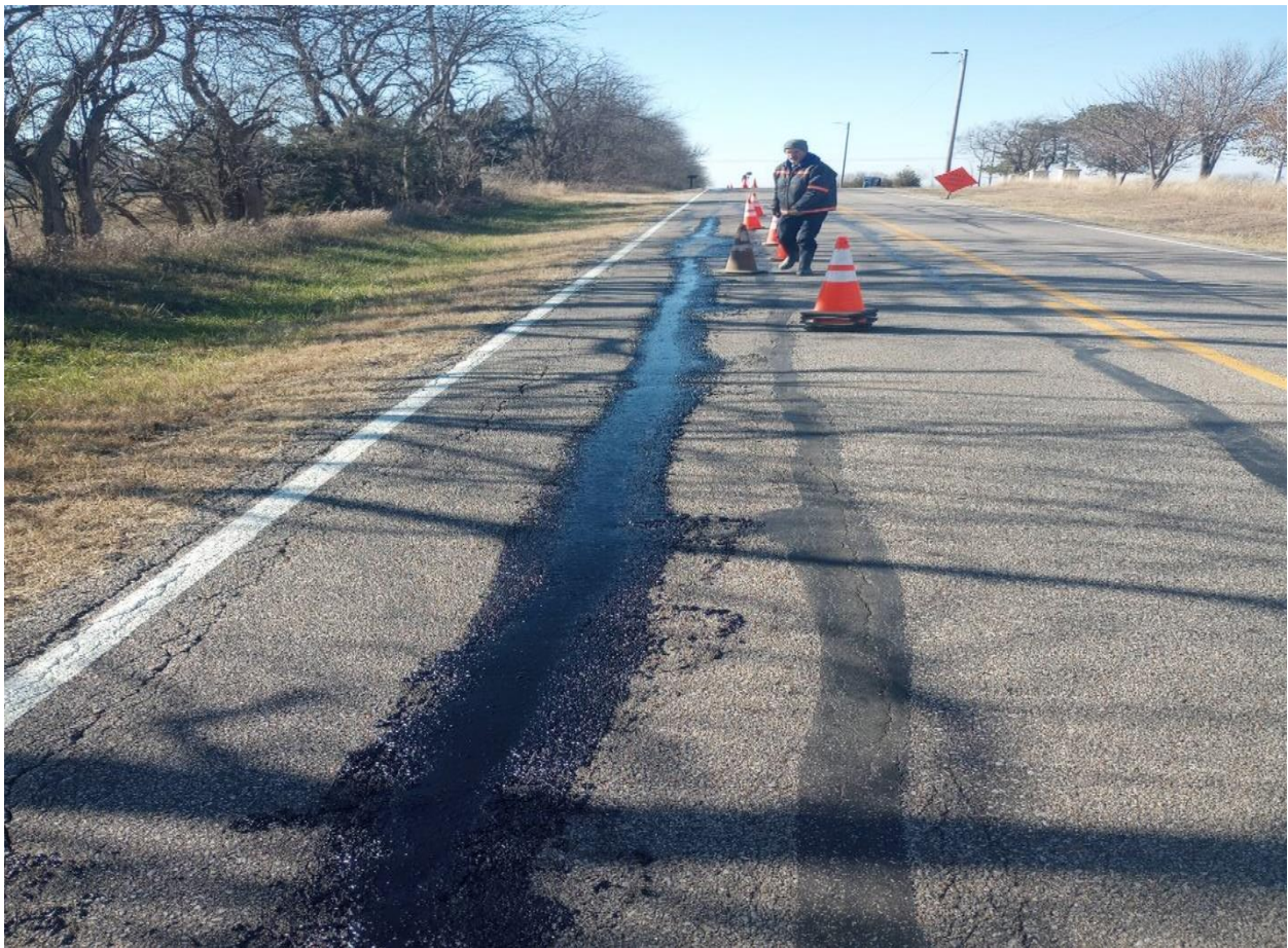
53 rd street repair
