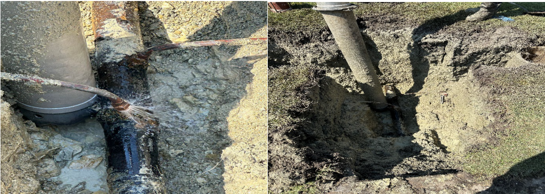
5800 block of Odessa 4" main with long 2 services that we replaced because of pipe damage.
