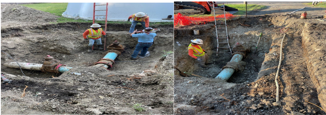
South Water tower replaced three valves.
