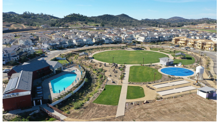
Post Construction Photo County of San Diego Harvest Park and adjacent private recreation center
