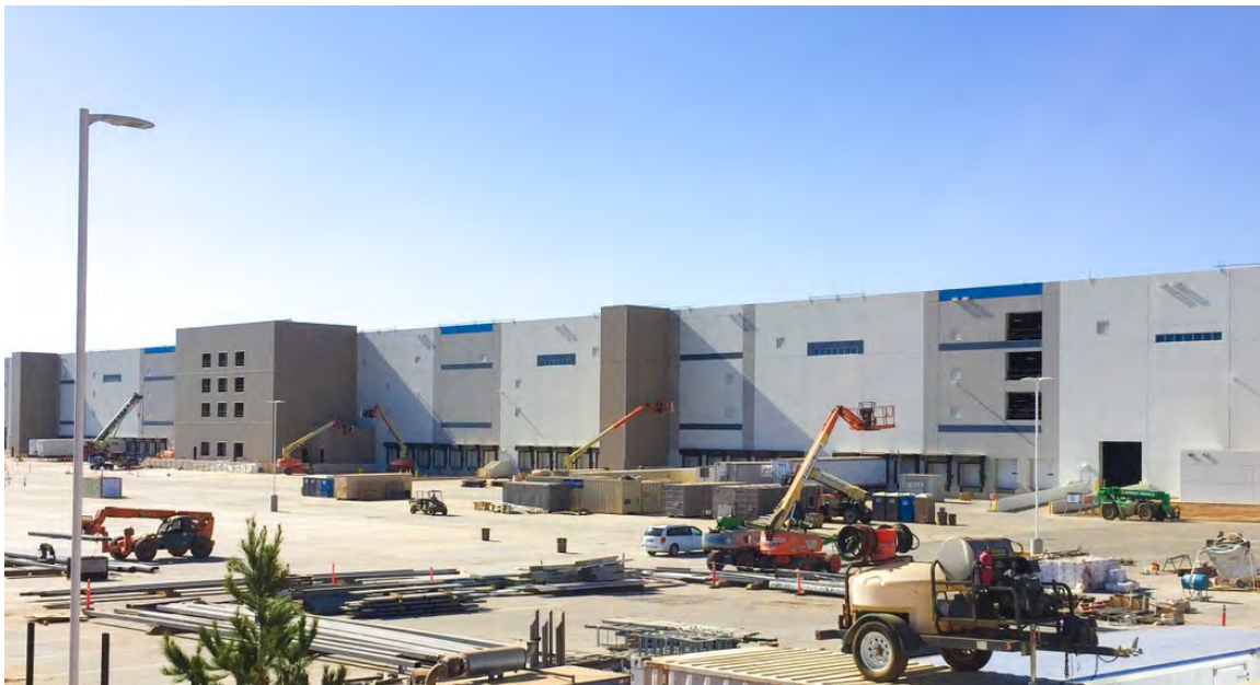
Beaumont’s Amazon warehouse during construction.
