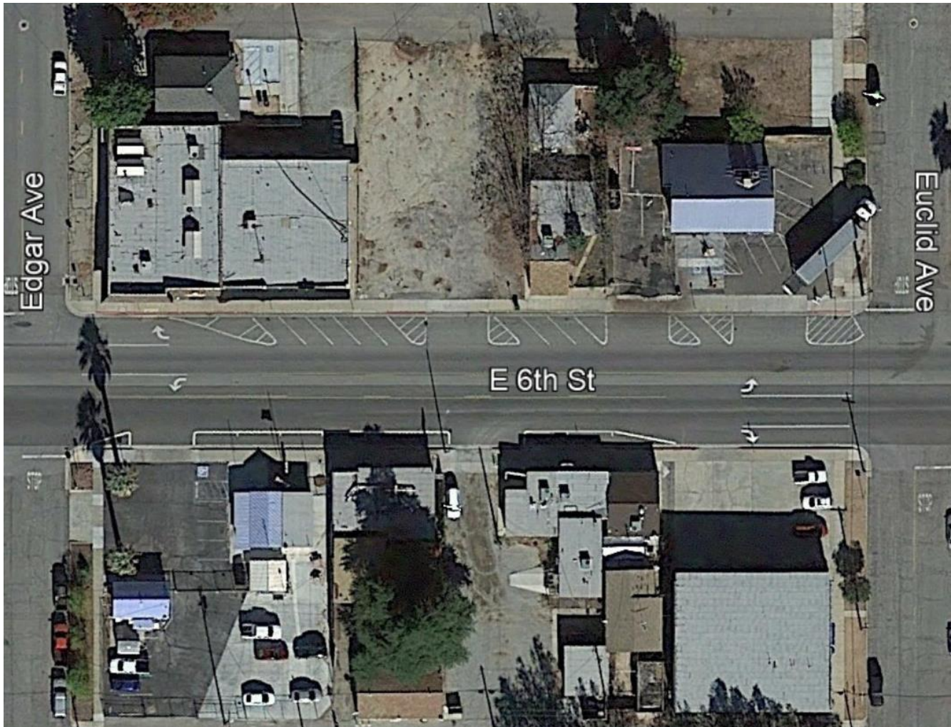
Figure 9: Striped On-Street Parking Stalls
