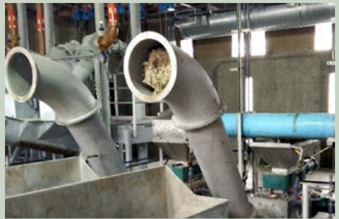
Rags and trash are flushed into the cutters, where grinding and washing dislodge fecal matter.
