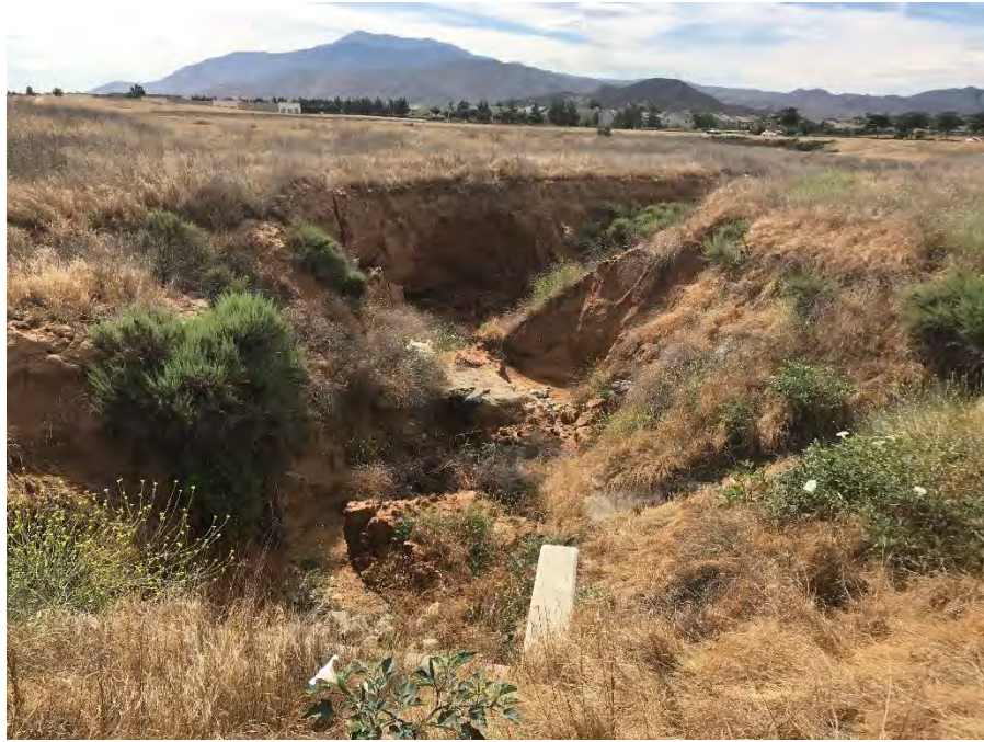
Photo 5 – Drainage B canyon connected to box culvert.
