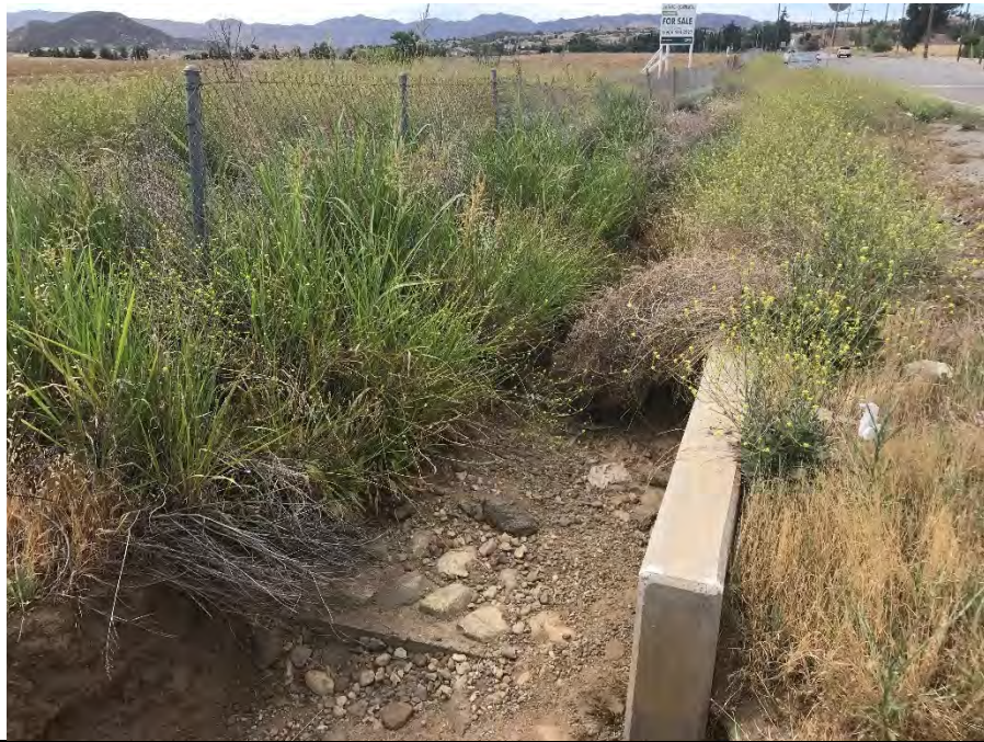
Photo 6 – Rushes associated with Drainage A. Section along Pennsylvania Ave.
