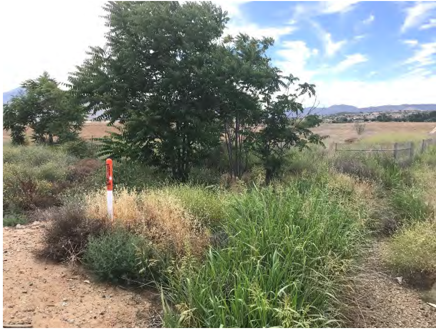
Photo 7 – Drainage A. Tree of Heaven and rushes/grasses growing near culvert
