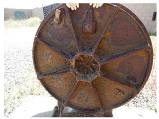
Heavy corrosion on underside of lid
