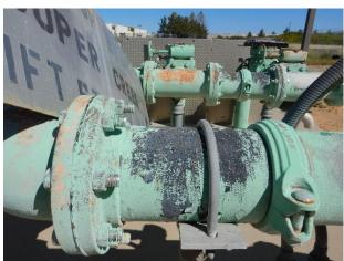
Factory coating evident through thinned coating (typical)
