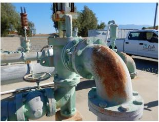
Surface corrosion typical throughout piping
