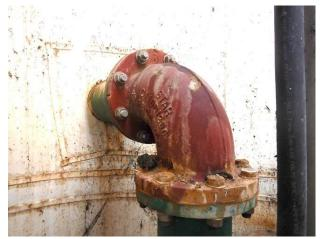
Pump discharge piping, minor corrosion at bolts/flanges
