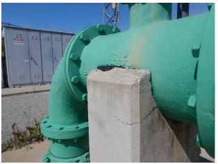
Cracking under Pump #1 pipe support
