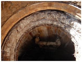
Non-mortared joints with exposed aggregate
