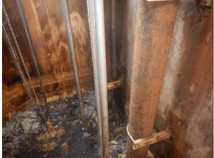
Surface corrosion typical throughout pump discharge piping
