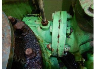
Pump #2 corrosion at bolts/flanges
