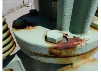
Corrosion typical where coating has flaked
