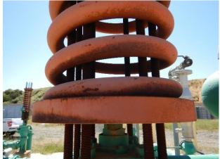
Corrosion at CAVs (closeup)
