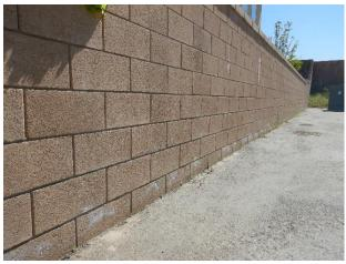
Efflorescence typical along bottom 0"-12"
