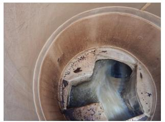
Bypass MH #2 interior, small tears within 3-ft of the bench
