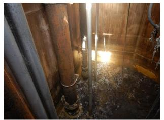
Surface corrosion typical throughout pump discharge piping
