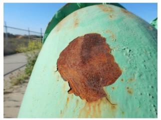
Surface corrosion (closeup)
