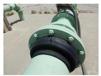
Cracking in rubber flexible couplings (typical)
