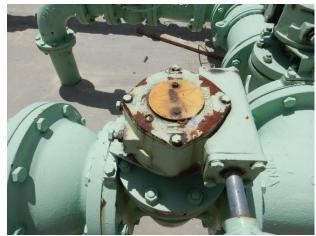
Minor corrosion at bolts, flanges, plug valves
