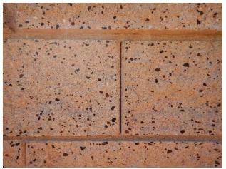
Missing mortar at vertical CMU joints (typical)
