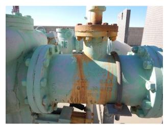
Corrosion staining from tap connection
