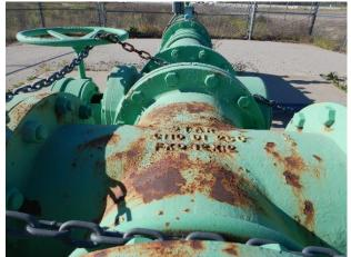
Surface corrosion typical throughout piping
