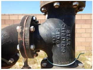
Minimal surface corrosion typical at flanges
