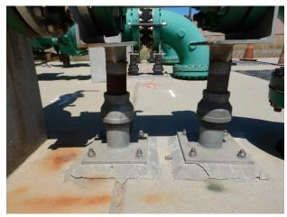
Cracking at pipe support concrete bases (typical)
