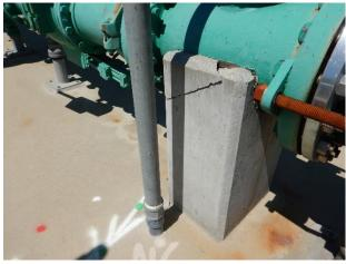
Cracked concrete pipe support (Pump 2)
