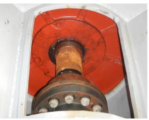
Corrosion on pump shaft (Pump 4)
