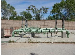
Aboveground piping, sagging in the center (Pump Assembly #3)
