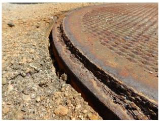
Bypass MH #3 (north) welded shut with corrosion
