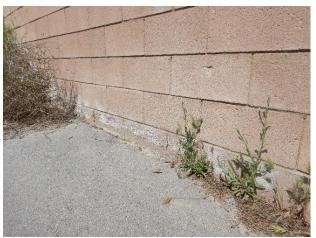
Spalling block (closeup)
