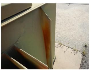
Surface corrosion on transformer
