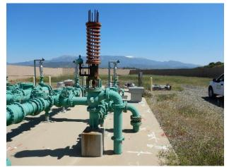
Corrosion at CAVs (typical)
