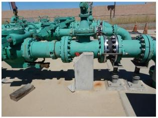
Cracked concrete pipe support (Pump 1)
