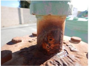
Corrosion at ARV tap connection (Pump 1)
