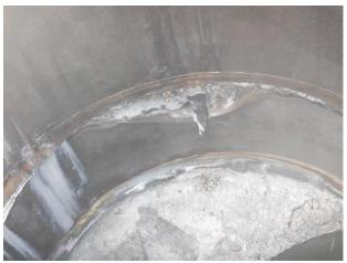
Liner disbonding from concrete (typical)
