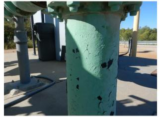
Coating peeling/flaking at riser sections (typical)
