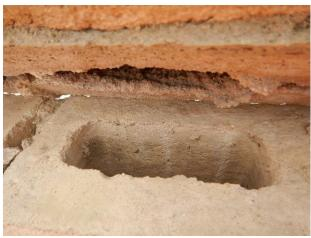
Missing grout inside of south wall
