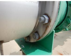
Dissimilar metal bolts/nuts used on SST pipe
