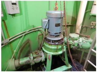
Pump #2, leak at pump/motor
