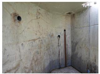
Corrosion staining on southwest wall
