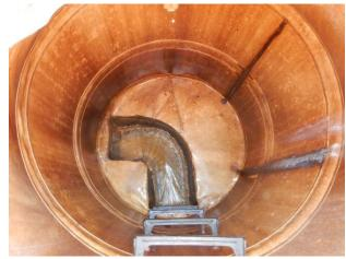
Bypass MH interior, pinholes in liner
