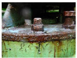
Pump #2 corrosion due to leak (closeup)
