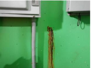
Corrosion where lined has failed (NW wall)
