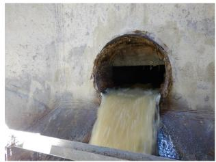
Influent pipe, heavy corrosion (closeup)
