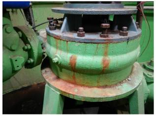
Pump #1 corrosion at bolts
