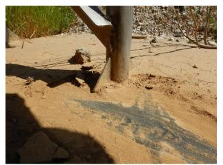
Cracking external rubber seals (typical)
