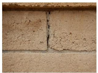
Mortared joints cracked with voids (typical)
