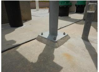
Concrete base for metallic pipe supports
