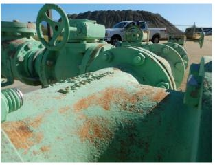
Surface corrosion typical throughout piping
