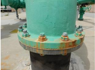
Corrosion typical at bolts/flanges
