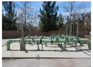
Aboveground piping, sagging in the center (Pump Assembly #1)
