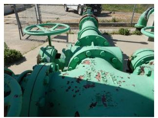
Cracked/peeling coating with corrosion typical throughout piping
