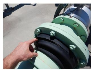
Cracking external rubber seals (typical)
