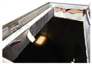
Liner disbonding at top of the structure
