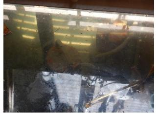
Sump pumps submerged, corroded
