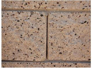
Missing mortar at vertical CMU joints (typical)
