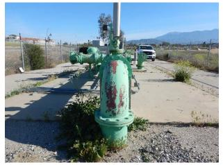
Surface corrosion typical throughout piping
