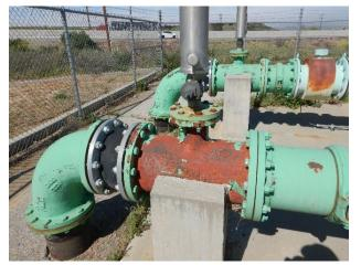
Surface corrosion typical throughout piping
