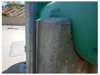
Cracking under Pump #2 pipe support
