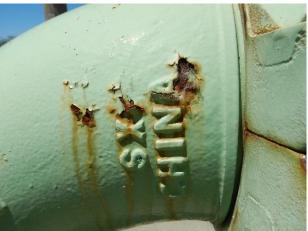
Corrosion typical where coating has flaked
