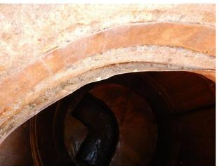
Bypass MH liner disbonding from cone
