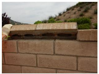
Masonry wall cap loose
