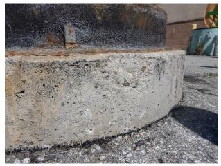
Exposed aggregate at wet well concrete collar
