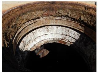
Bypass MH exterior, corrosion at rim
