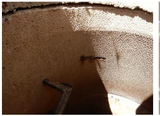
Spiral reinforcement breaching concrete
