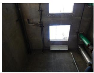
Efflorescence on ceiling around openings
