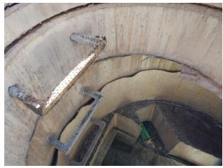
Liner disbonding from the concrete
