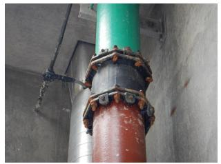
Corrosion typical on hardware at flexible couplings
