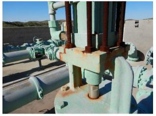
Corrosion at CAVs (typical)
