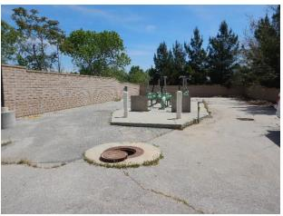
Cracking in asphalt leading from major equipment
