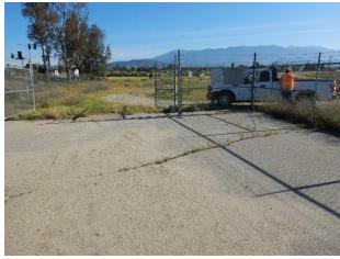
Cracking in asphalt near entrance
