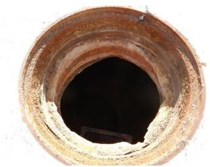
Bypass MH exterior, corrosion at rim
