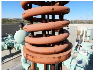
Corrosion at CAVs (typical)
