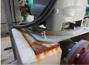
Corrosion at pump/motor base plates (Pumps #1-2)
