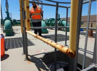
Dry well access swing gate corroded throughout
