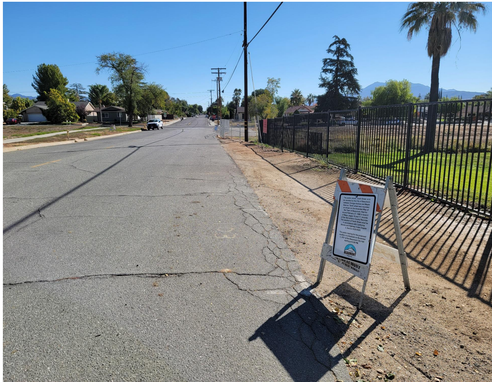
Tenth Street – Looking East
