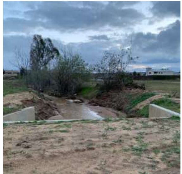
Figure 8. Existing Culvert/Storm Drain North of E. 2 nd St.
