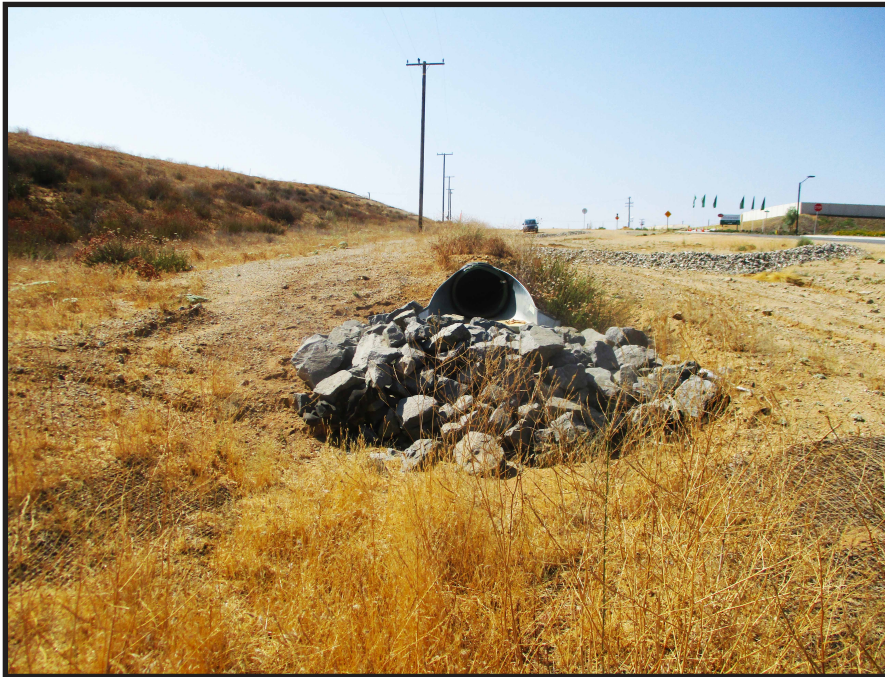
PHOTOGRAPH 6 - Southward view of offsite drainage ditch that the onsite ravine flows toward. Riversidean sage scrub occurs on the western Project Site manufactured slope (red boundary).
