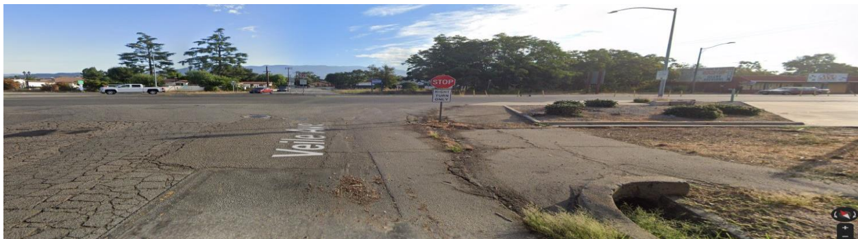
Figure 3 - Existing Traffic Control Devices and Striping at Northbound Veile Ave
