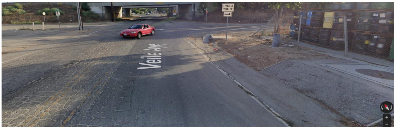
Figure 10 - Existing Traffic Control Devices and Striping at Northbound Veile Ave
