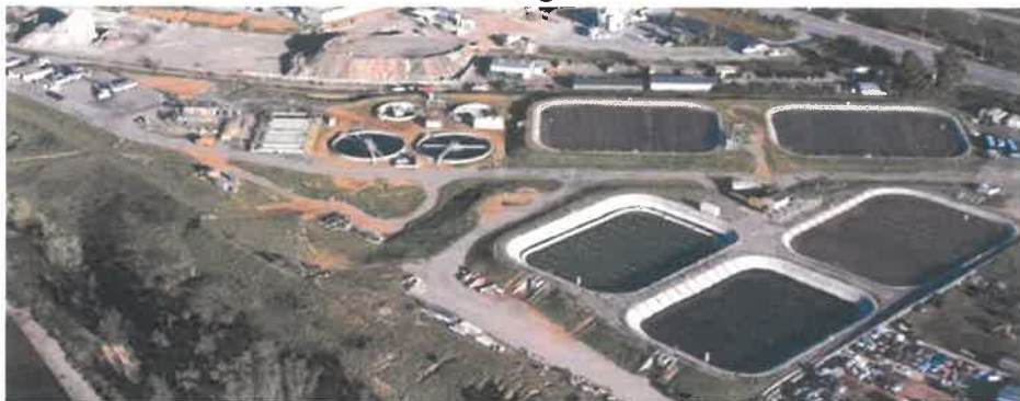
Figure 1 – City of Beaumont Wastewater Treatment Plant
