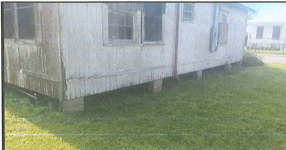
Photo 032625 unevenness of cinder blocks supporting structure
