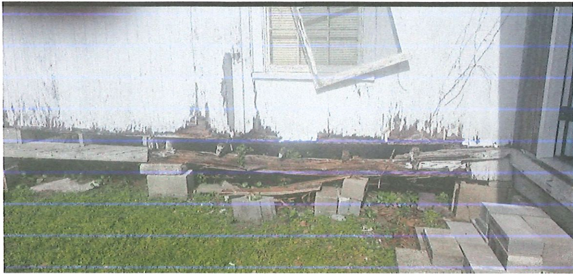
Photo 032625 deterioration of foundation and horizontal beam
