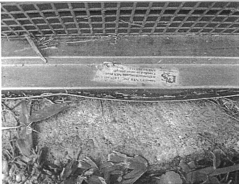
Photo Three Caption: Flood Vent Information (Smart Vent rated for 200 square feet each)
