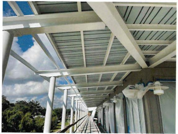
Painting is complete at all steel roof structure and framework of the upper-level walkway.
