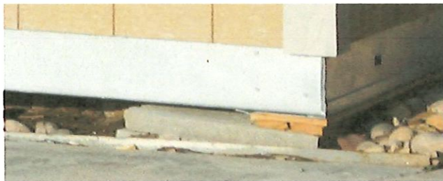
Figure 2 - Close-up of leveling with blocks & shims
