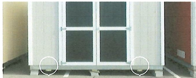
Figure 3 - Display building with wood skids beneath the floor joists
