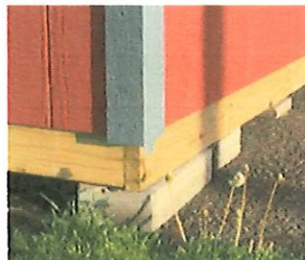
Figure 2 - Close-up of leveling with blocks & shims
