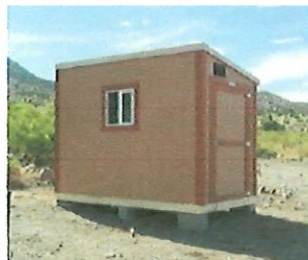
Figure 2 - Close-up of leveling with blocks & shims
