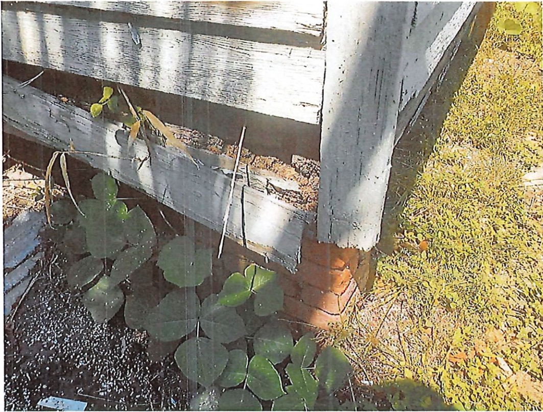
Photo 091223 exterior wall damage from weathering and termites.
