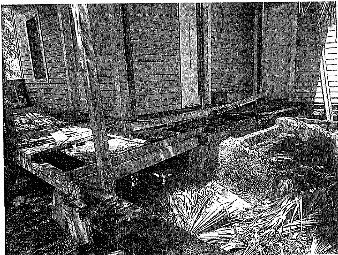
Photo 091223 deterioration of foundation elements
