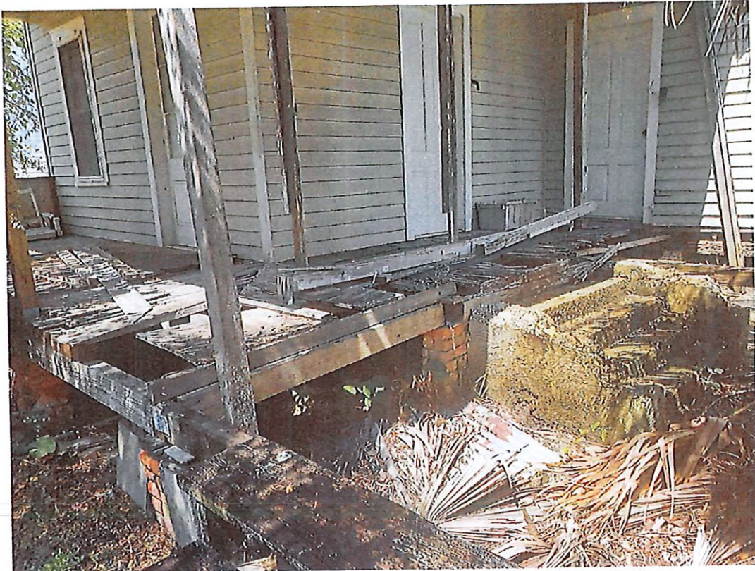
Photo 091223 deterioration of foundation elements
