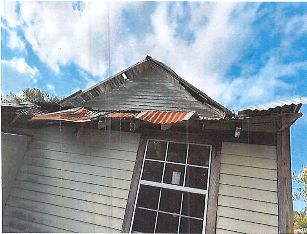
Photo 092023 a non existent load path from roof to exterior walls and indications of settlement. Sincerely
