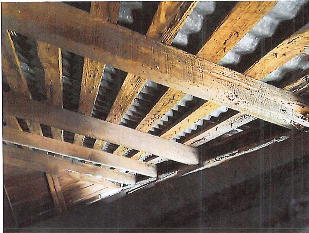
Photo 091223 rafter and purlin damage and a non-existent load path from the roof to the exterior walls
