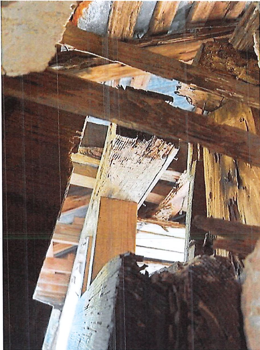
Photo 092023 roof deterioration from weathering and termites of rafters, cross bracing and purlins
