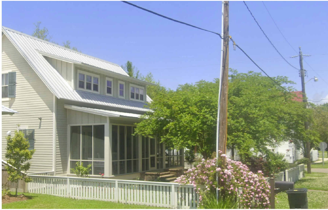
EXISTING HOME - VIEW FROM HANCOCK ST.
