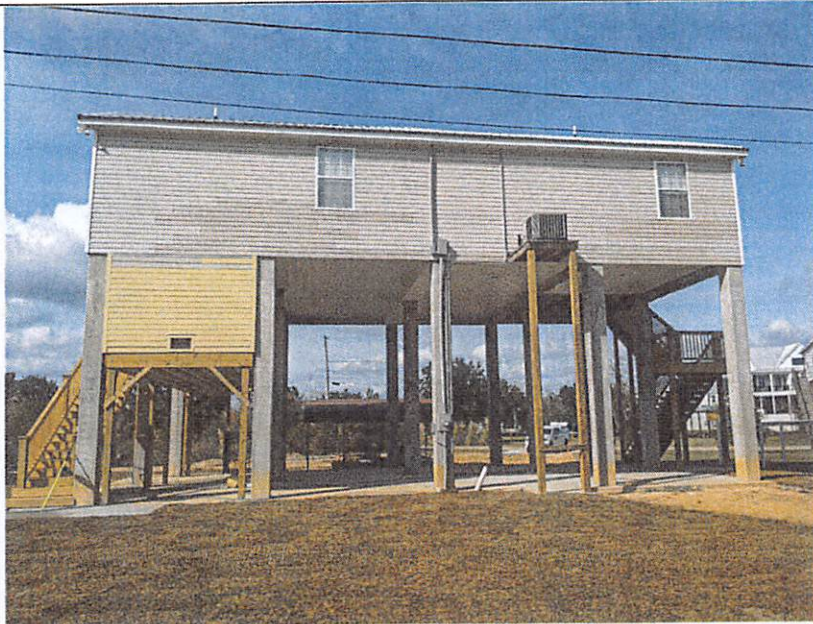
Photo Two Caption: South Side showing HVAC Equipment Clear Photo Two
