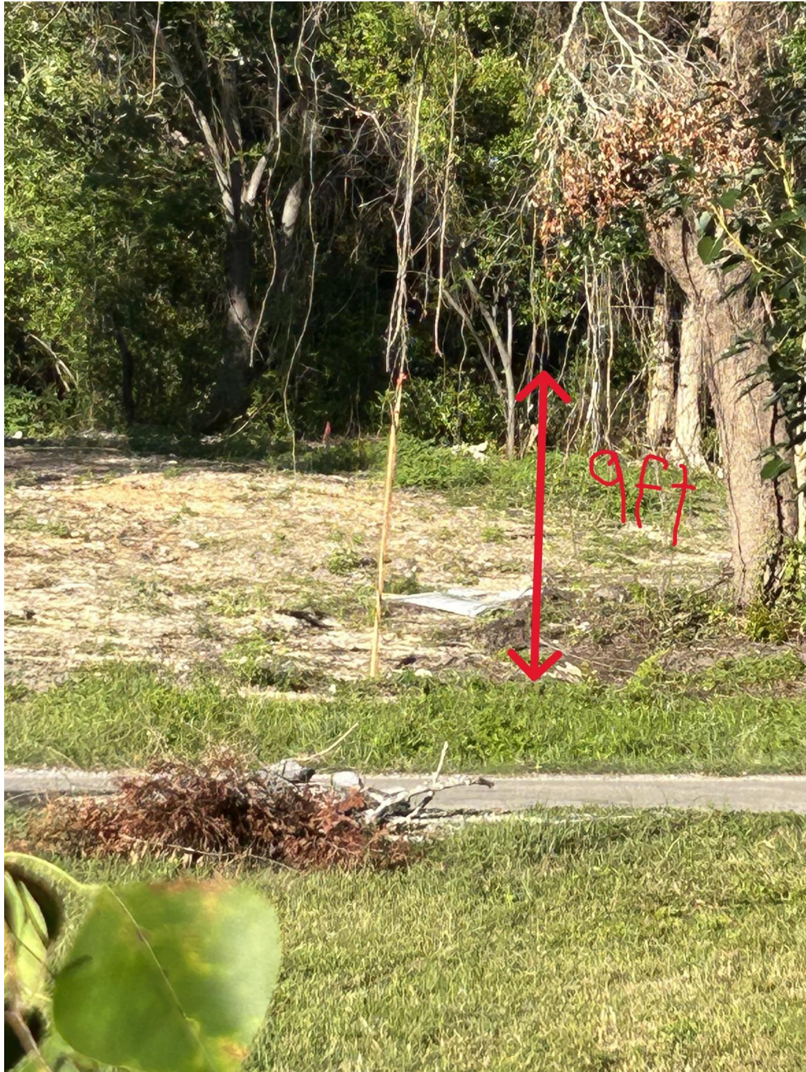
Figure 2: Same stake indicating 9-8ft of fill, but from the perspective of looking across Webster Street. Arrow is closer to actual retention wall, approximately 6 to 10ft from Oak in the picture.
