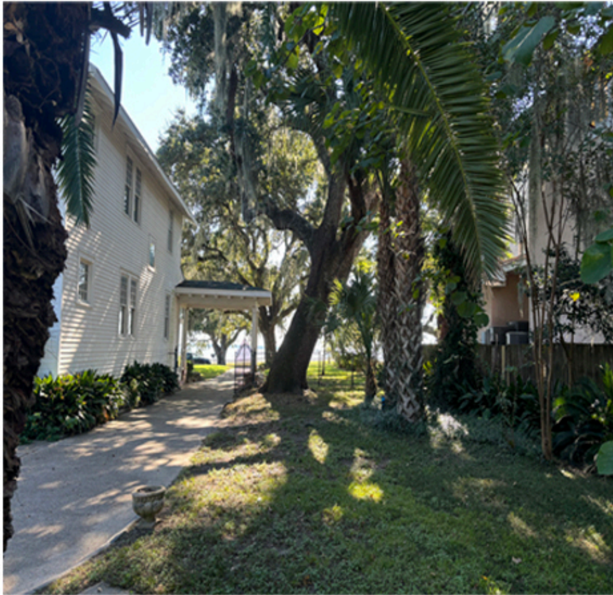
SOUTH SIDE OF HOUSE
