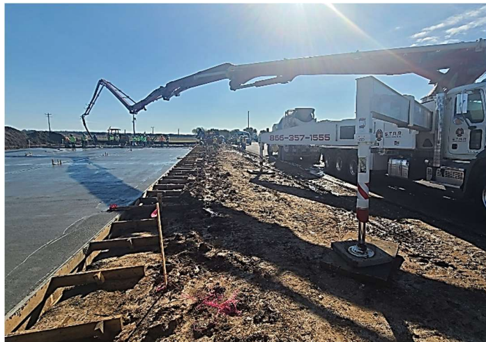
Figure 2 – Concrete placement of the foundation
