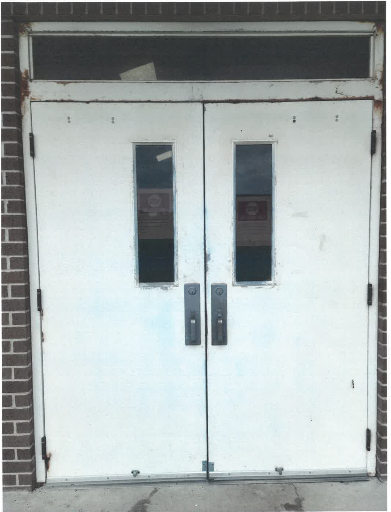
South Exterior Entrance to Dining room
