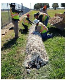
Figure 1- Installation of Filter Dam
