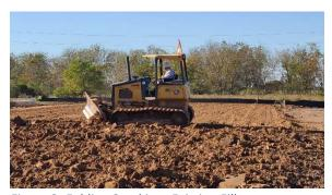
Figure 3- Folding Sand into Existing Fill
