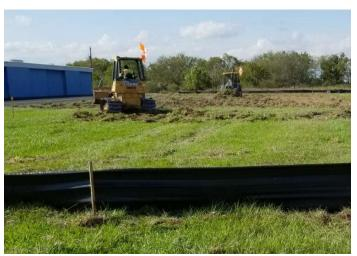
Figure 2 - Stripping topsoil for grading
