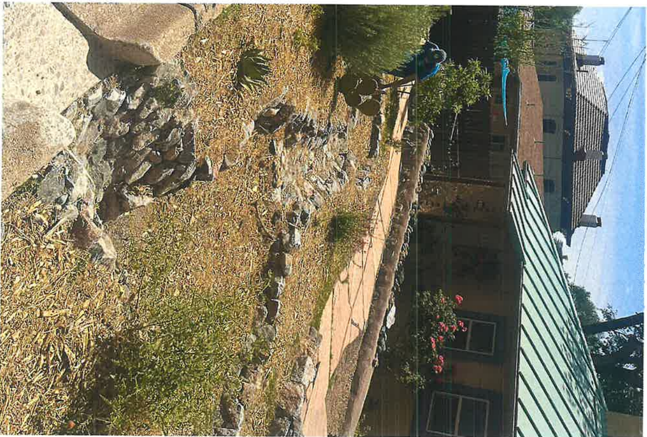
Curb cut, bioswale and basin complex in Silver City constructed by Asher Gelbart, Green Energy Now, that will allow stormwater to irrigate the landscape and reduce flooding in streets during storm events.
