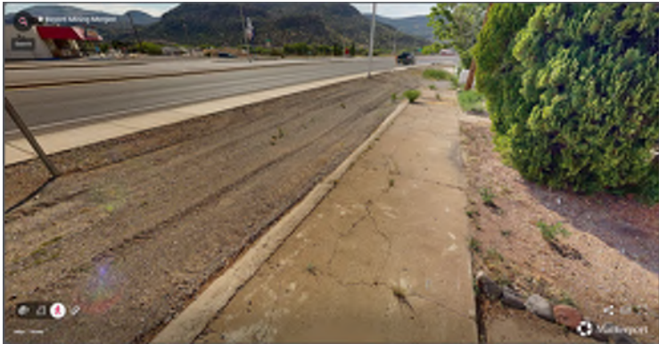
Project North: Building Front (NE)
