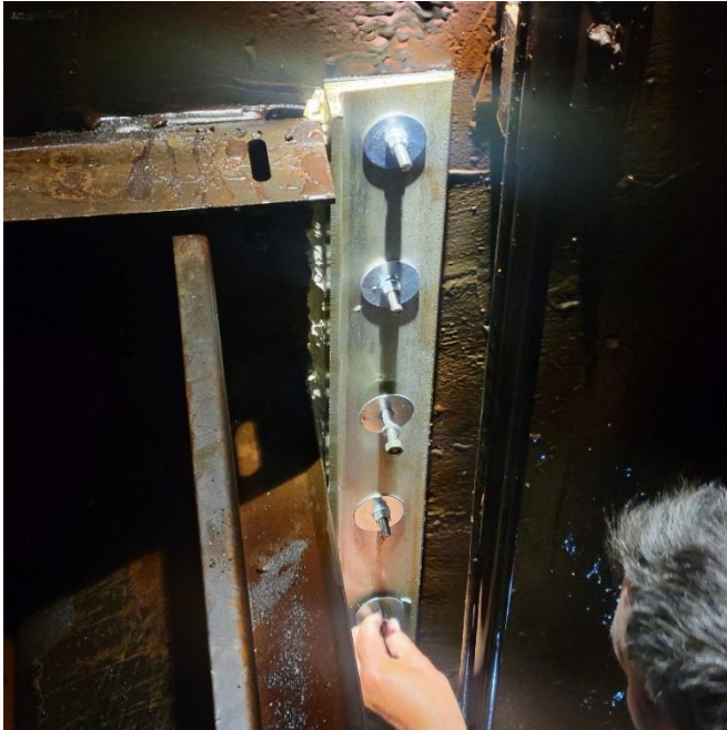
3. Reinstalling washers, lock washers, and nuts on studs.
