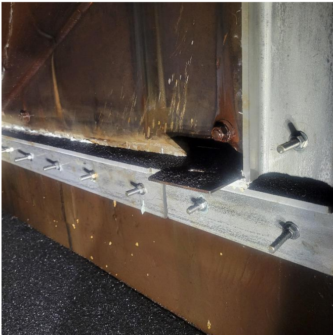
2. Example of angle bracket installation.
