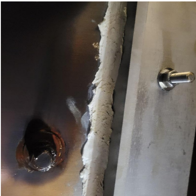
4. Example of Waterweld application.
