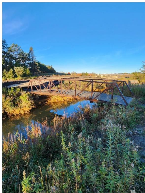
The bridge superstructure is in good condition with no noticeable defects in the steel portion. The timber plank are in fair to good condition with some minor deterioration starting. The concrete abutments are showing signs of severe deterioration along the top of the backwall and abutment seat,
