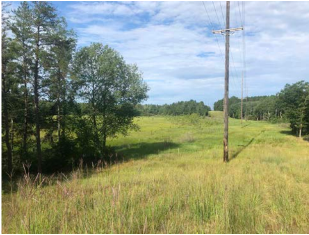
Existing east-west utility corridor, looking west.
