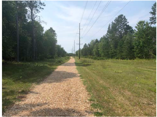
Existing Woodchip Trail, looking west along the east-west utility corridor.
