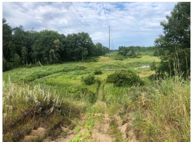
Existing east-west utility corridor, looking west over Pike Creek, adjacent wetlands, and tamarack stand.
