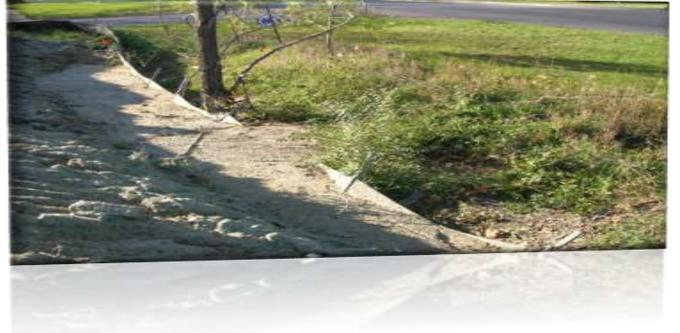
Improper perimeter control allowing for sediment to discharge offsite
