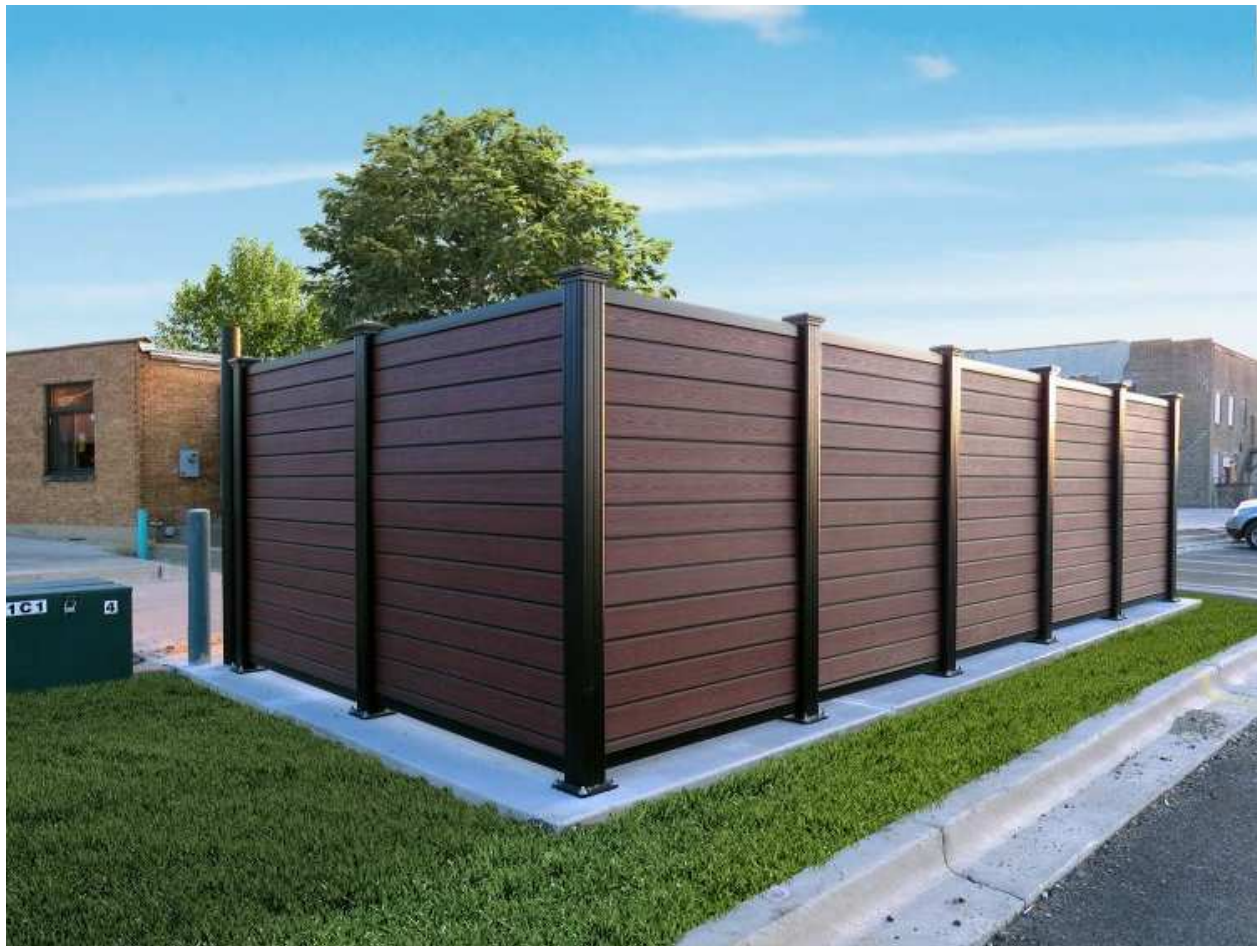
Dumpster Enclosure - Rear/Side View
