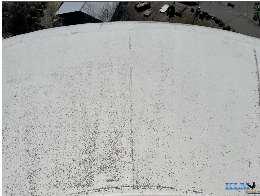
Photo No. 20 Roof plate coating conditions
