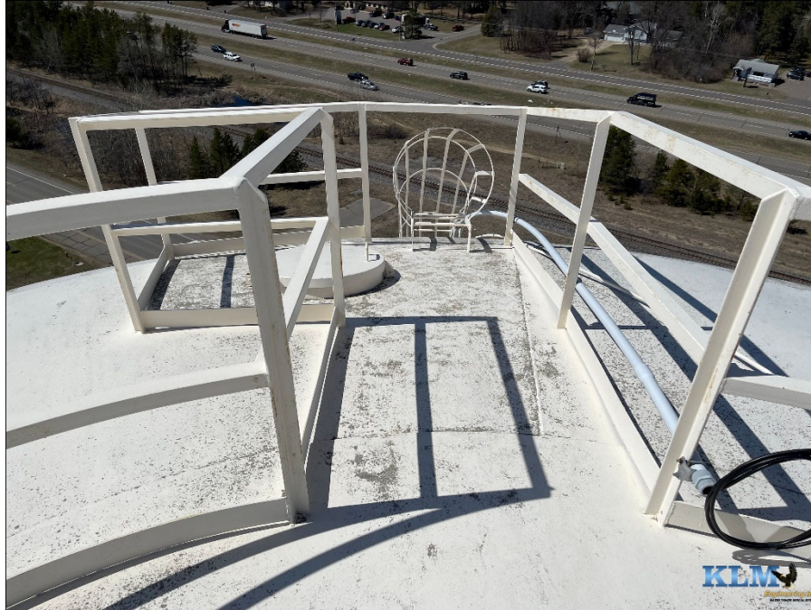
Photo No. 21 Roof handrail
