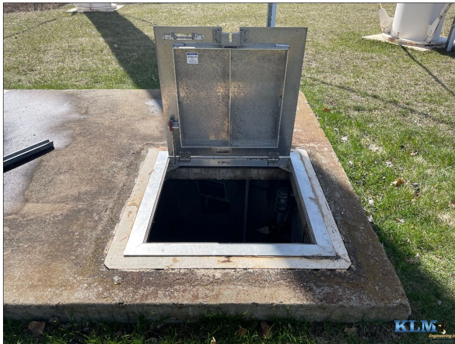
Photo No. 38 Valve pit manway
