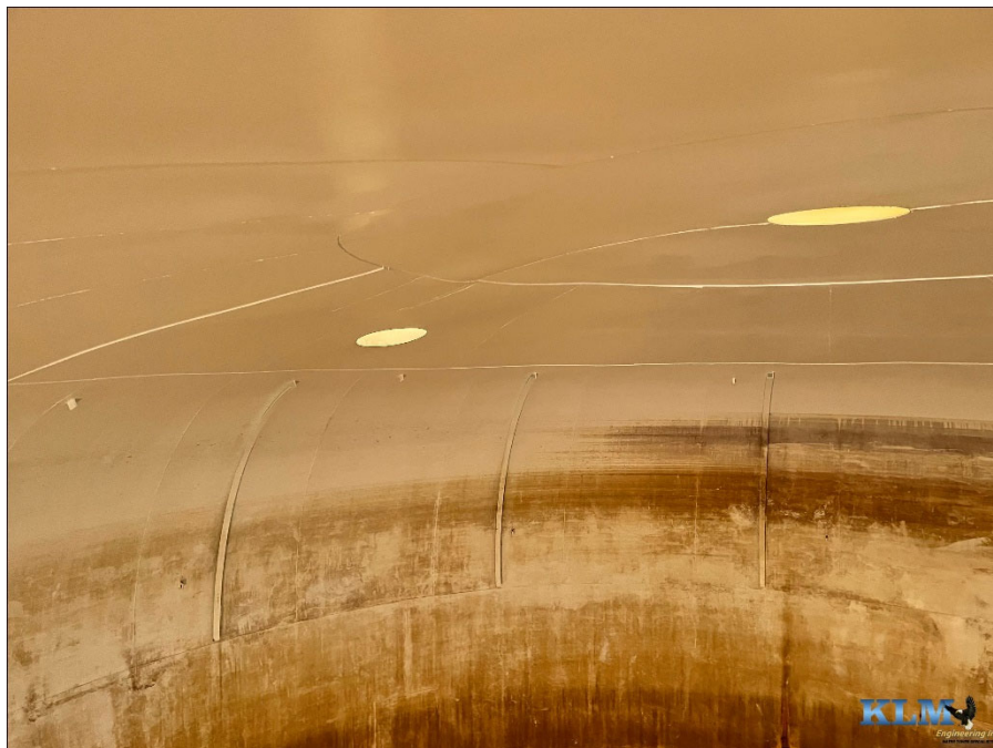
Photo No. 4 Condition of roof plate coatings
