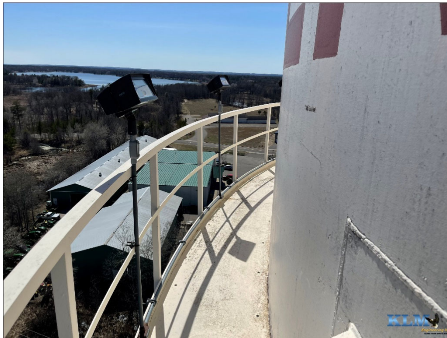
Photo No. 26 Balcony and handrail
