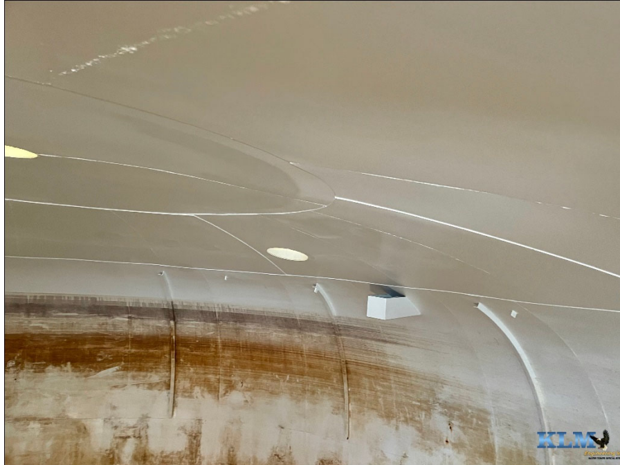
Photo No. 3 Condition of roof plate coatings Overflow weir box visible
