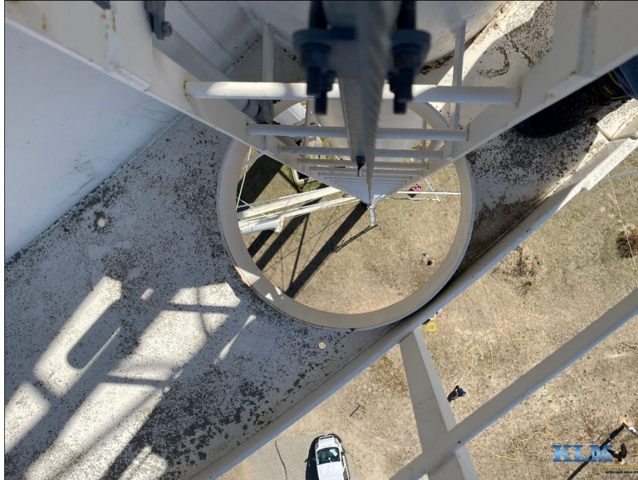
Photo No. 29 Column ladder
