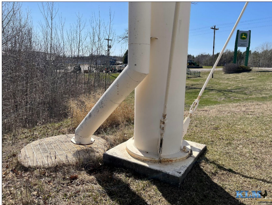
Photo No. 36 Overflow pipe and grating
