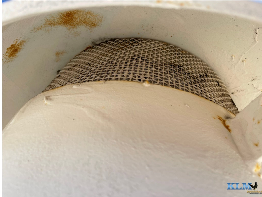
Photo No. 17 Condition of finial vent
